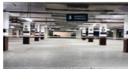
100% LED LIGHTS INSTALLATION
