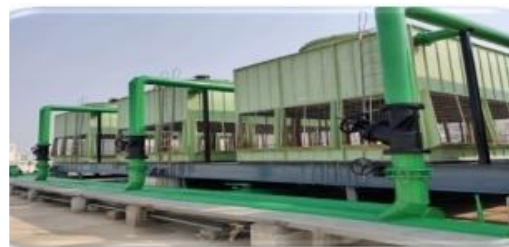
COOLING TOWER UPGRADATION
