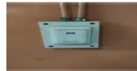
BASEMENT EXHAUST INTERGRATION WITH CO SENSOR
