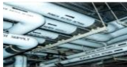
CHILLED WATER RING MAIN LINE INTERCONNECTION
